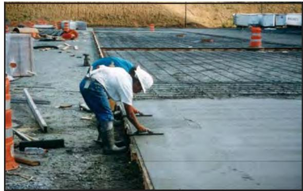
Future ACI documents will recommend that construction joints be saw cut 1" (25 mm) after the concrete has hardened and a crack develops. This saw cut creates a reservoir for a joint filler, reveals any inherent weakness in the formed joint edge due to lack of densification, and makes all joints look the same. The use of a 1/8" (3 mm) radius edging tool on the first pour creates a guideline for the saw to follow.
