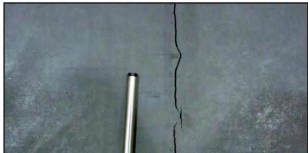
*The timing of the filler's installation is critical. Filling joints too early after slab placement (or before temperature draw down and stabilization in freezer/cooler rooms) can result in filler adhesion loss and separation from the joint walls, potentially leaving the joint edges exposed to impact and deterioration.*
