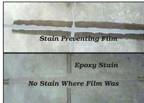
*The use of a stain preventing film can reduce or eliminate slab surface staining from epoxy/polyurea filler overfill. Other stain prevention methods include applying soap or wax.*
