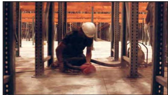
To compensate for low adhesion, fillers must be installed full depth in saw cuts. By filling full depth the bottom of the cut provides support for the filler when loads are imposed. Compressible backer rod should never be used at the base of saw cut joints because it negates the solid support provided by the cut bottom. If it is necessary to "choke off" the bottom of a saw cut to prevent material loss, dry bagged silica sand may be used in accordance with the filler manufacturer's data.
