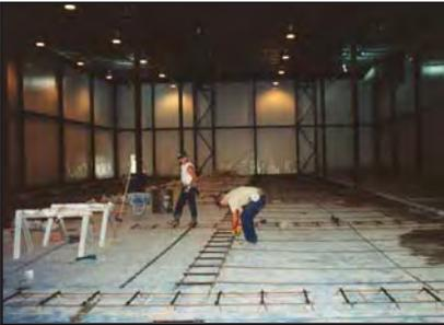
When round or square dowels are used at contraction joints, placement directly under the subsequent joint is critical.
