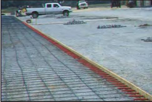
*It's critical that dowels be set at the proper depth and at a 90° angle from the joint to avoid slab damage.*
