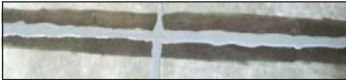
Always Overfill Joints (Surface shown with SPF Film)
