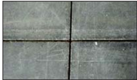
Minor edge chipping is not unusual on new floors to be filled. Chips wider than 1/16th" (2mm) should be “squared off” prior to filling.
