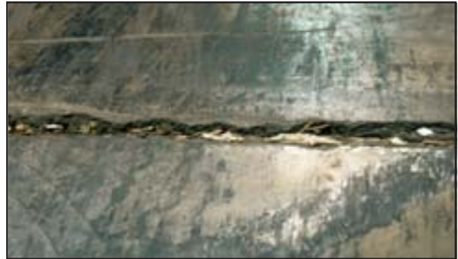
Deteriorated joints create an interruption in the continuity of the floor surface, leading to operational slow-downs and increased vehicle maintenance costs.
