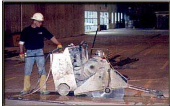
Traditional “wet cut” saws require sufficient slab cure to support the saw's weight.
