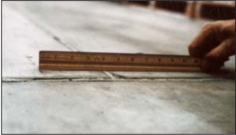
Slab edge curl can occur when the top of the slab dries at a significantly faster rate than the slab bottom. A curled edge creates an impact point at the joint, and left untreated will likely spall under material handling vehicle traffic (below).
