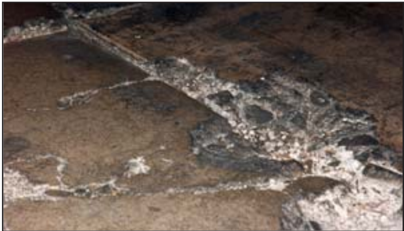
Slab edge curl can occur when the top of the slab dries at a significantly faster rate than the slab bottom. A curled edge creates an impact point at the joint, and left untreated will likely spall under material handling vehicle traffic (below).
