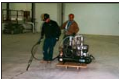
Polyureas, due to their fast gel times, require the use of dual-component pumps to install. Epoxies can be dispensed manually through bulk caulking guns or through a dual-component pump as well.
