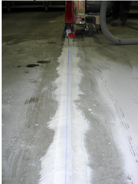
Snap Line Over Original Joint
