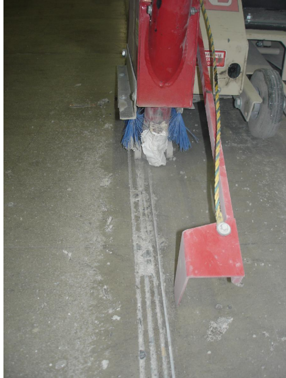
Saw Cut Lines Behind Spall
