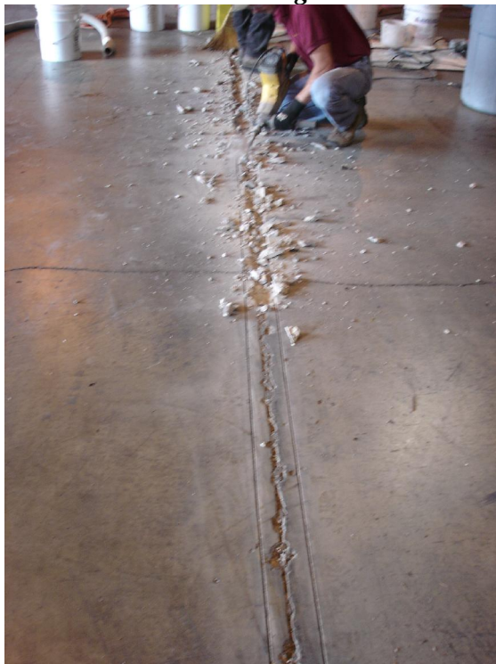
Remove Remaining Concrete
