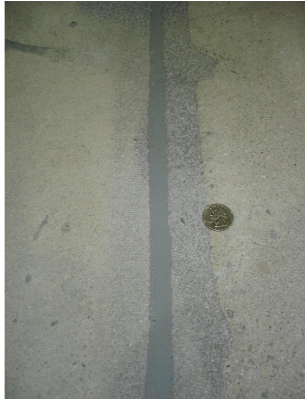
Restored Joint Condition
